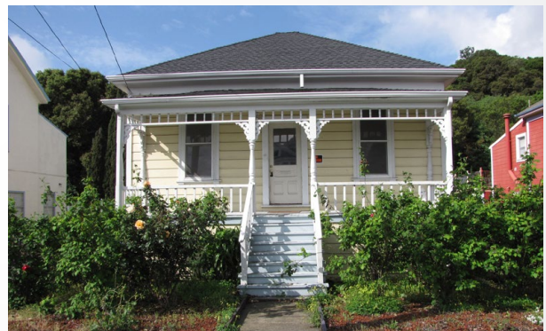
Original 1 story building
